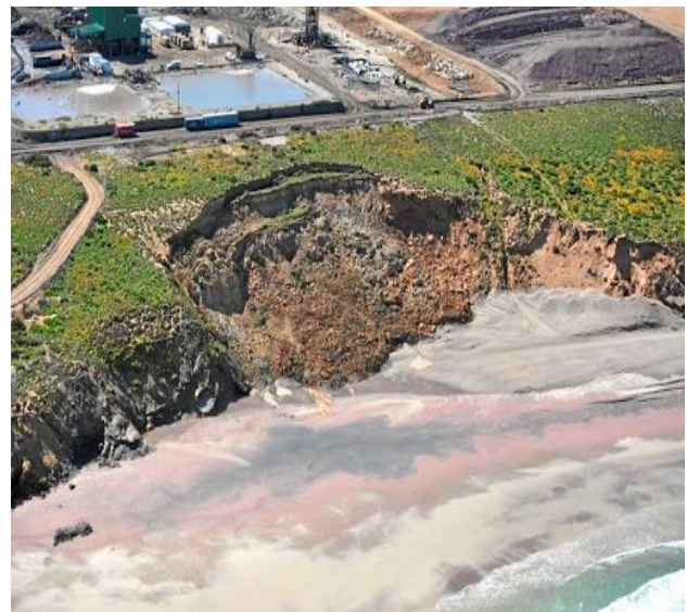
The cliff has collapsed. The mining company denies any responsibility
