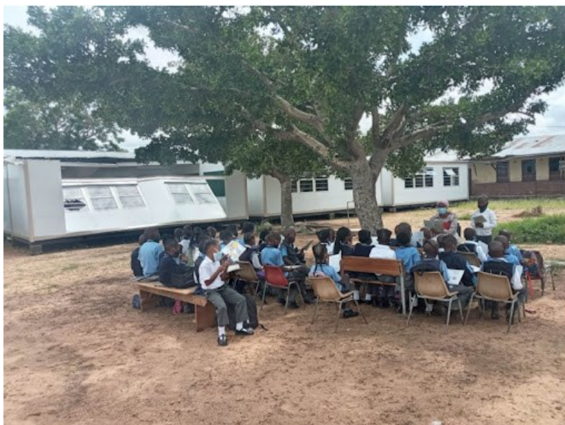
Children learning under a tree with dilapidated prefabricated buildings in the background
